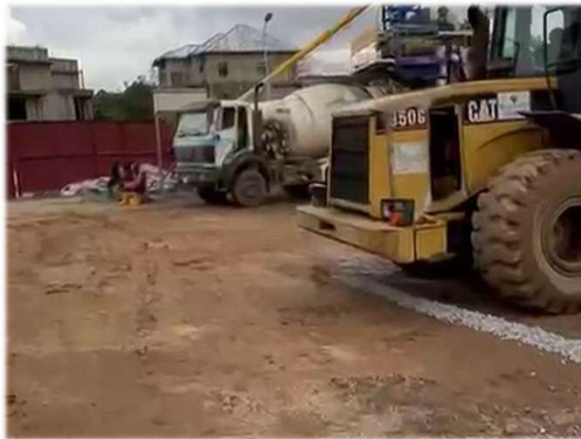
Concrete-production and construction equipment
