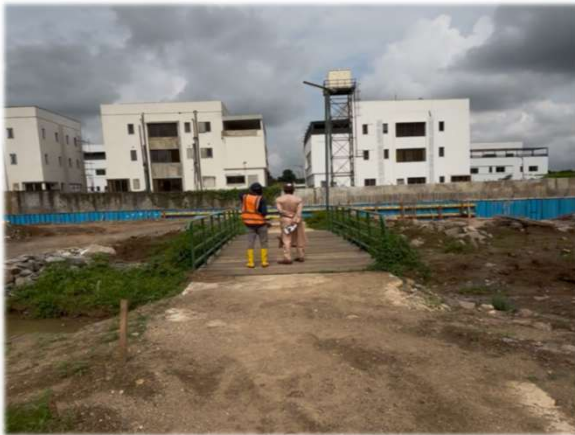
Site access and early infrastructure activity
