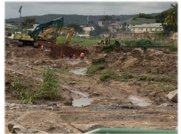
Earthmoving equipment and material handling
